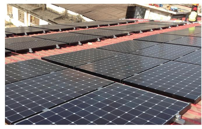
Type: 318W Mono-Crystallite Back-Contact Technology without Light Induced Degradation (LID) Effect
